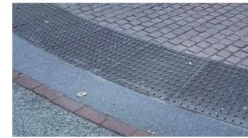
① Bump Out with Flush Curb and TWSI
