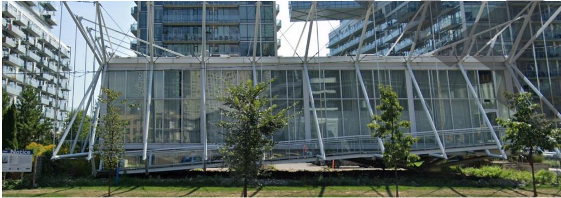
Steel and wire cable spider with 'sails'
