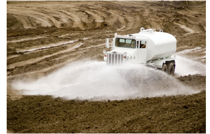
Construction site watering for dust
