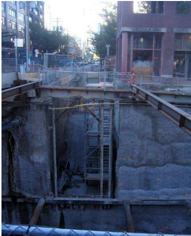
Exhibit 2-57: Examples of open cut construction for below grade sections
