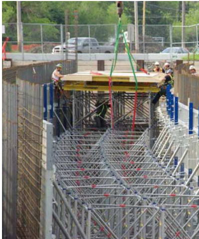
Exhibit 2-57: Examples of open cut construction for below grade sections
