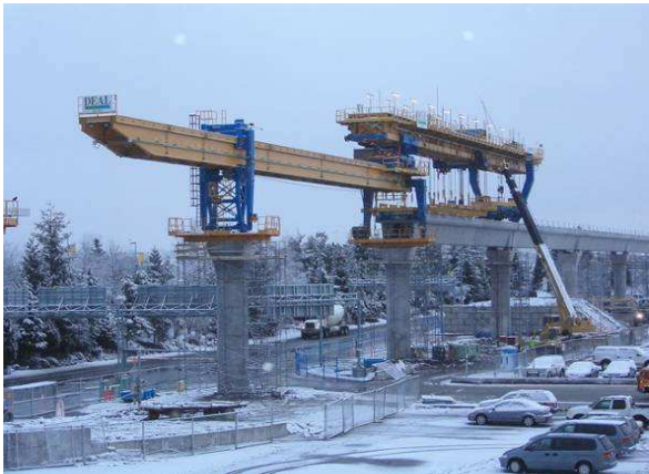
Beams can be assembled in segments on site and put into place using precast segmental construction method.
