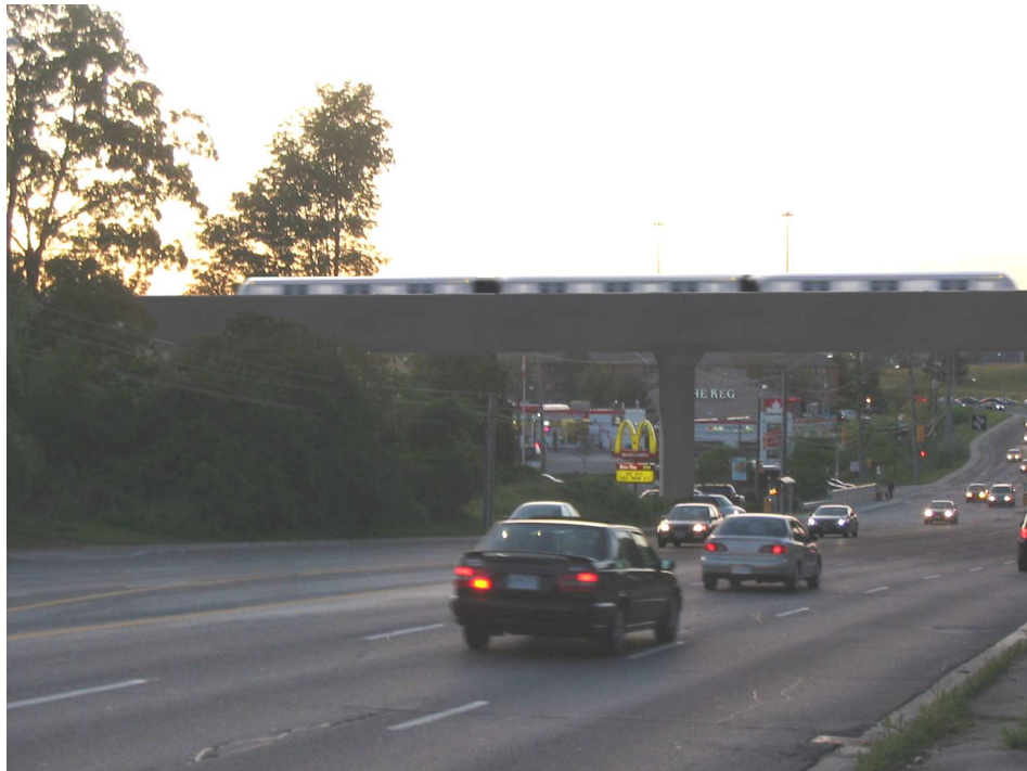
Exhibit 2-21: Elevated structure across Markham Road with columns in middle of road
