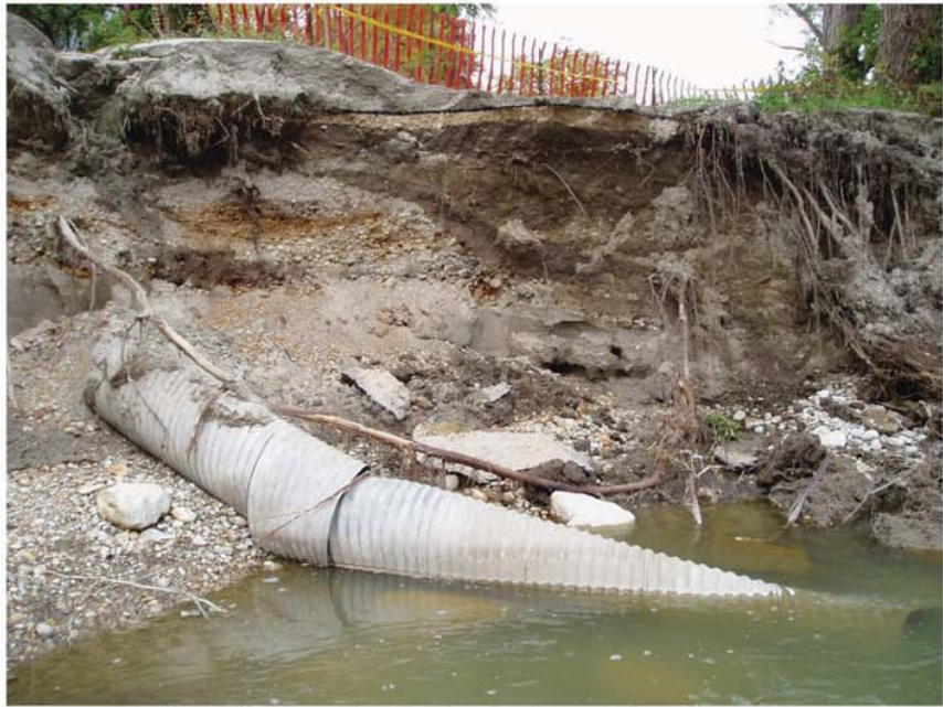
Photo 3. Exposed and undermined watermain and conduit.
