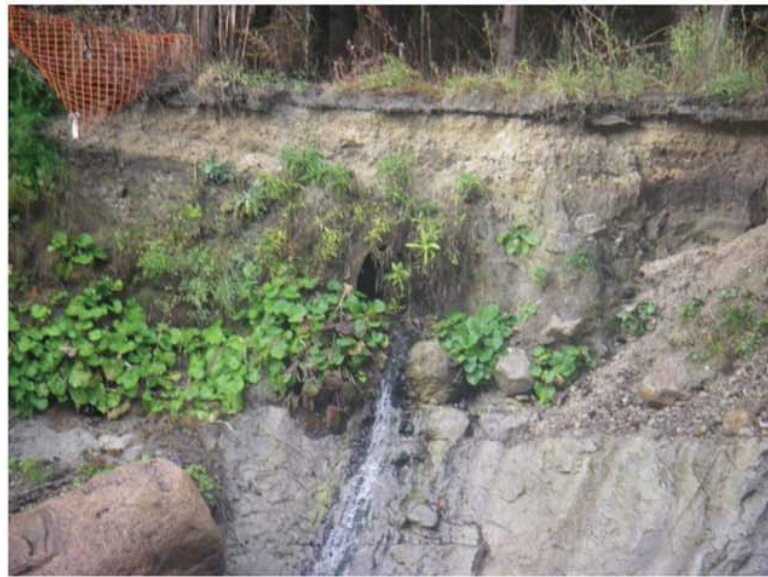
Photo 1. Elevated storm sewer outlet and erosion downstream of the pedestrian bridge.
