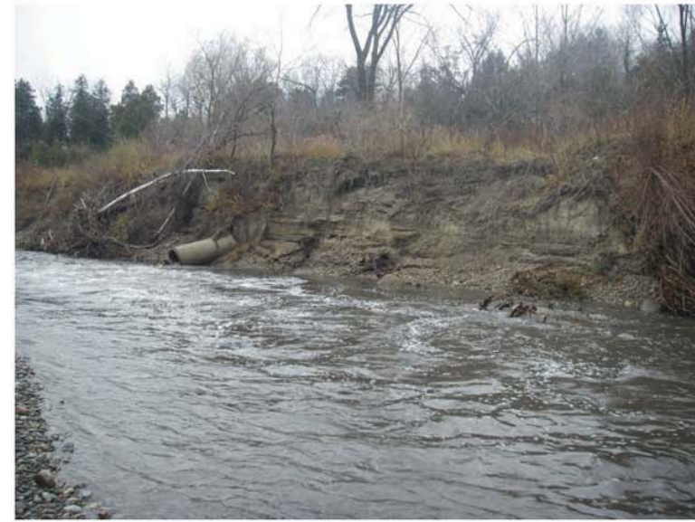
Photo 3. Bank erosion and exposed concrete pipe downstream of Morningside Avenue.
