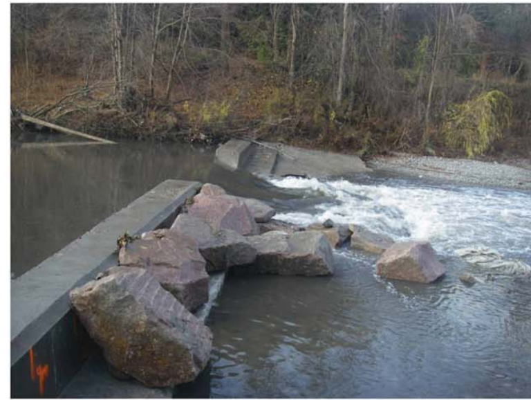
Photo 4. The weir upstream of Morningside Avenue.
