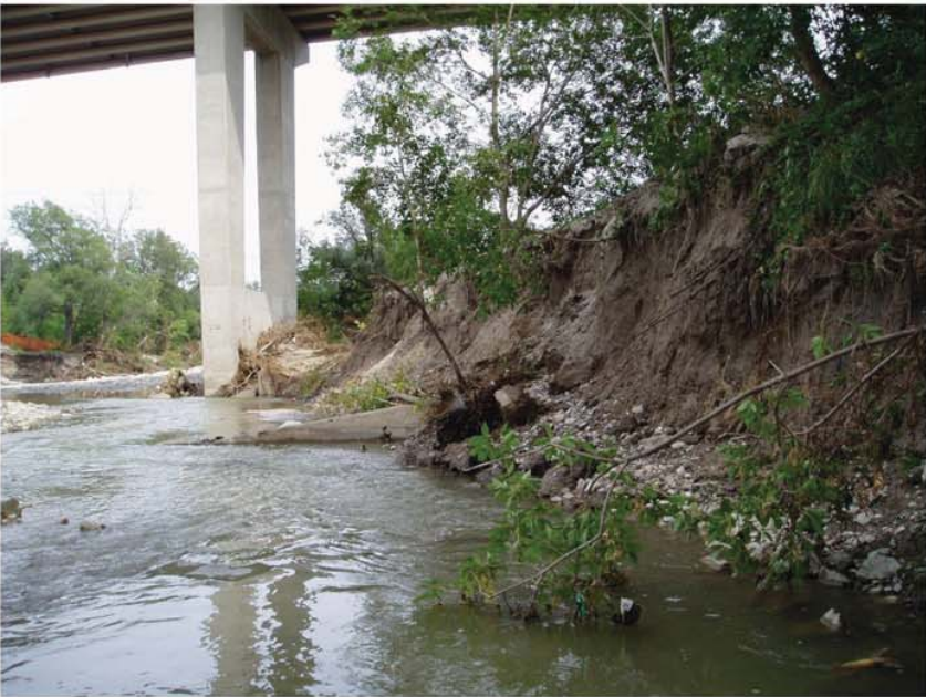
Photo 2. Exposed bridge pier and eroded bank.
