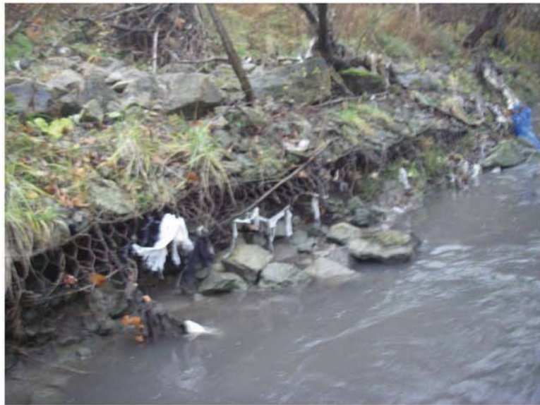
Photo 6. Failed gabion baskets upstream of Morningside Avenue.
