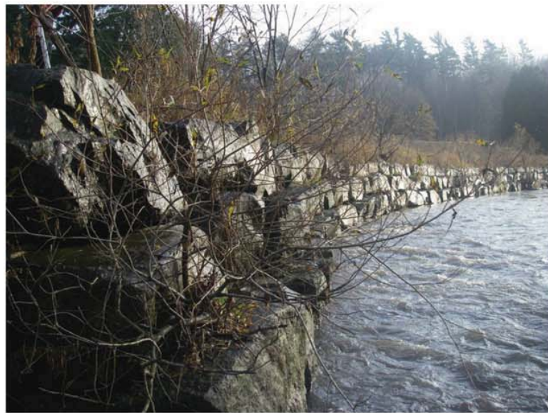
Photo 2. Armour stone wall downstream of Morningside Avenue.
