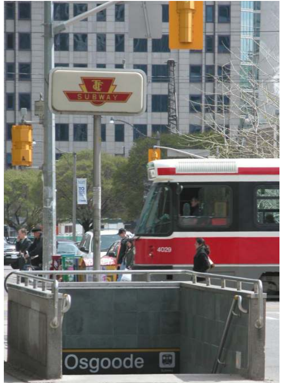
Existing Open Entrance
